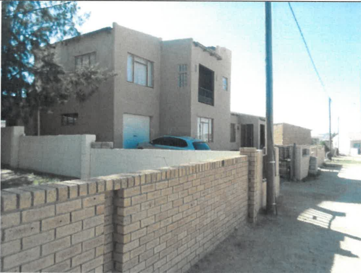
Figure 19: Maildrops done along Kerk Street.
