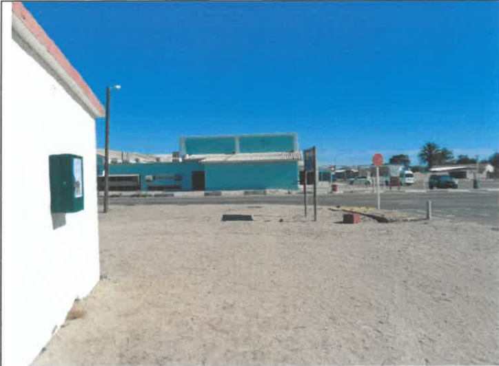
Figure 13: A3 Poster placed against an existing building, located approximately 14m south-west of the site. Looking in a south-western direction.
