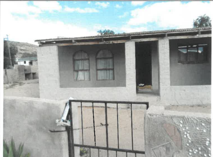
Figure 38: Maildrop done at residential dwelling along Omdraai Street
