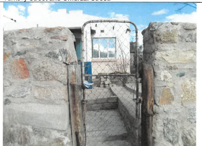
Figure 30: Maildrop done at residential dwelling along Omdraai Street.
