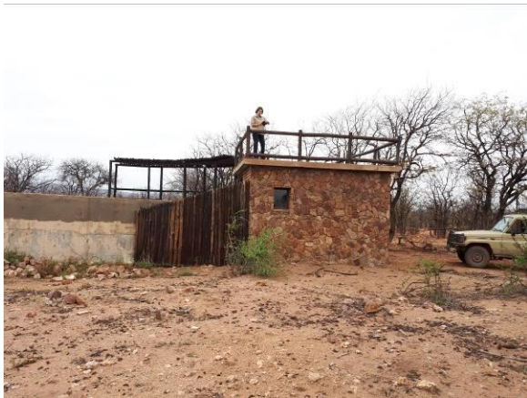
Existing reservoir and building on site
