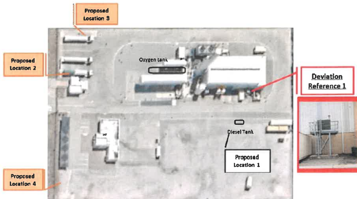
Figure 7. Locations of Diesel Tanks as reviewed by Major Risk Installation Assessment. The initial proposed location one is highlighted in white with all secondary locations highlighted in orange. Proposed locations 2 and 3 were submitted as the proposed diesel tank locations as depicted in Figure 4.
