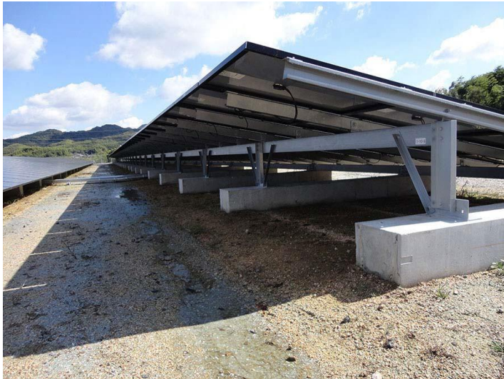
FIGURE 5: CAST CONCRETE FOUNDATION (SOLAR POWER PLANT BUSINESS, 2013)
