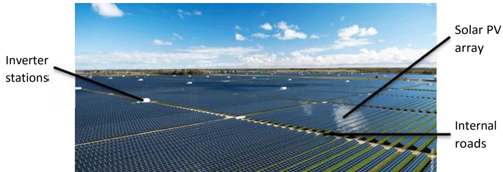
FIGURE 1: TYPICAL LAYOUT OF A SOLAR PV ENERGY FACILITY (THE MILLION SOLAR ROOF INITIATIVE – SOLAR SALVATION OR SOLAR SCAM? CALIFORNIA PV SOLAR FARMS – A BITTER HARVEST!, 2014)
