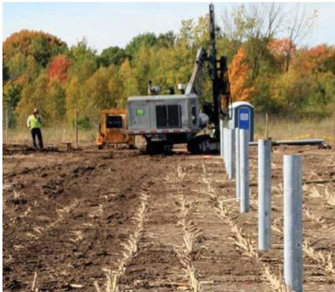
FIGURE 6: RAMMED / DRIVEN STEEL PILE (SOLARPRO, 2010)
