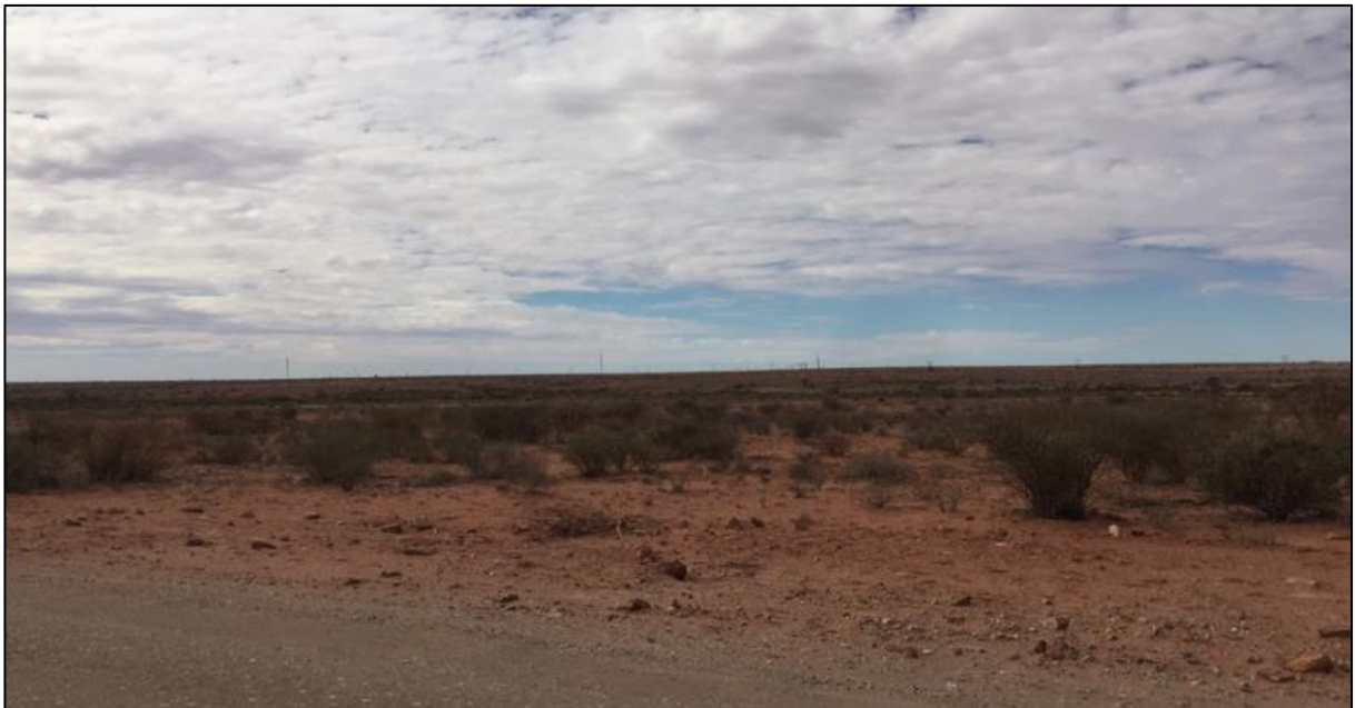
Figure 16: Survey Point 16 photograph taken to the southeast from the gravel road access to the under construction Sirius Solar PV Project One facility.
