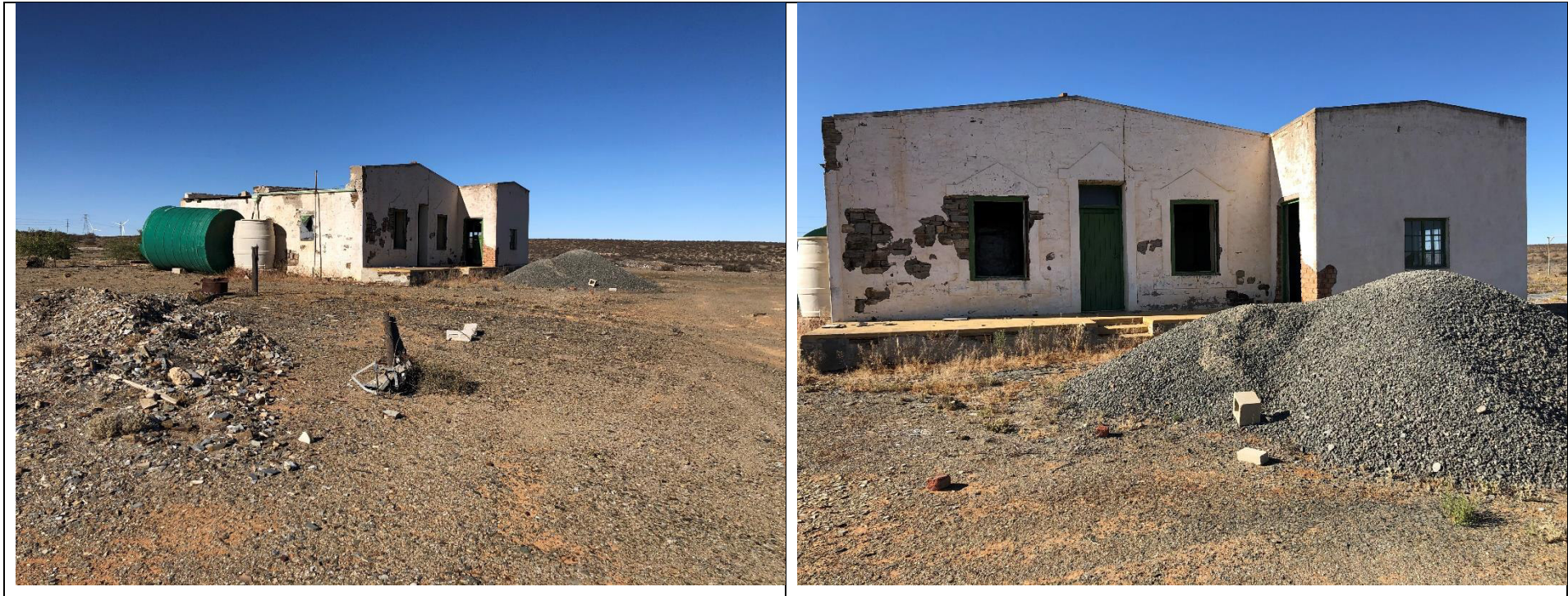
Figure D.2: Photos of the structure located at NSD 1
