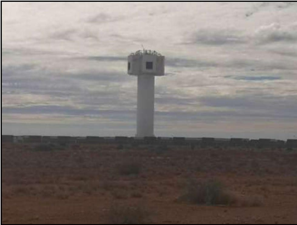
Photograph 1.14: Abengoa Khi Solar 1 CSP
