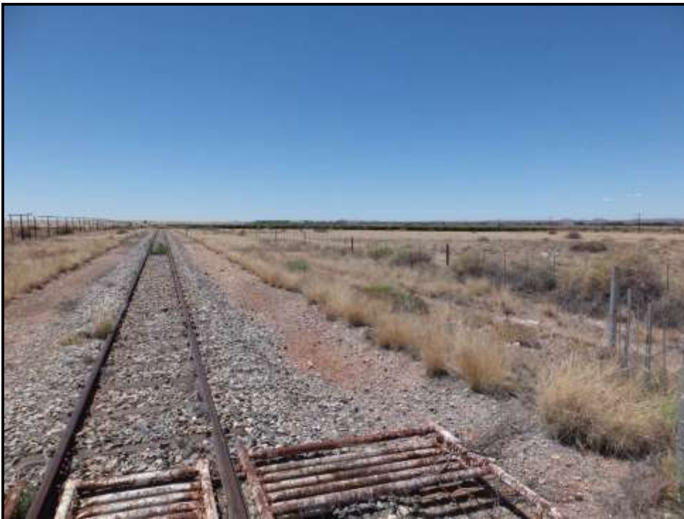
Photograph 1.2: Rail way line to the south of the site adjacent to N14
