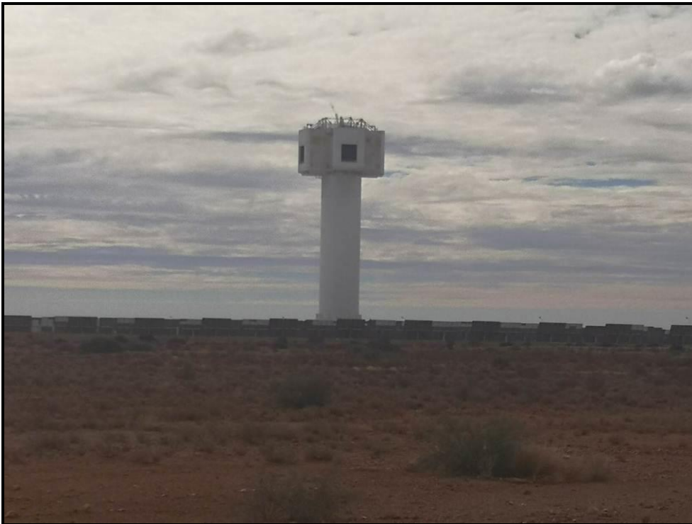
Photograph 1.14: Abengoa Khi Solar 1 CSP
