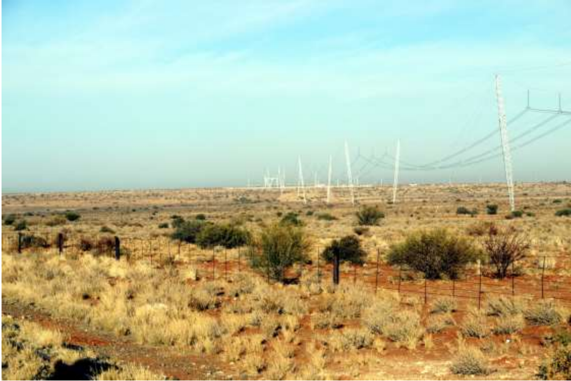
Plate 1, Existing Upington Main Transmission Substation viewed from the Lutzputs Road.
