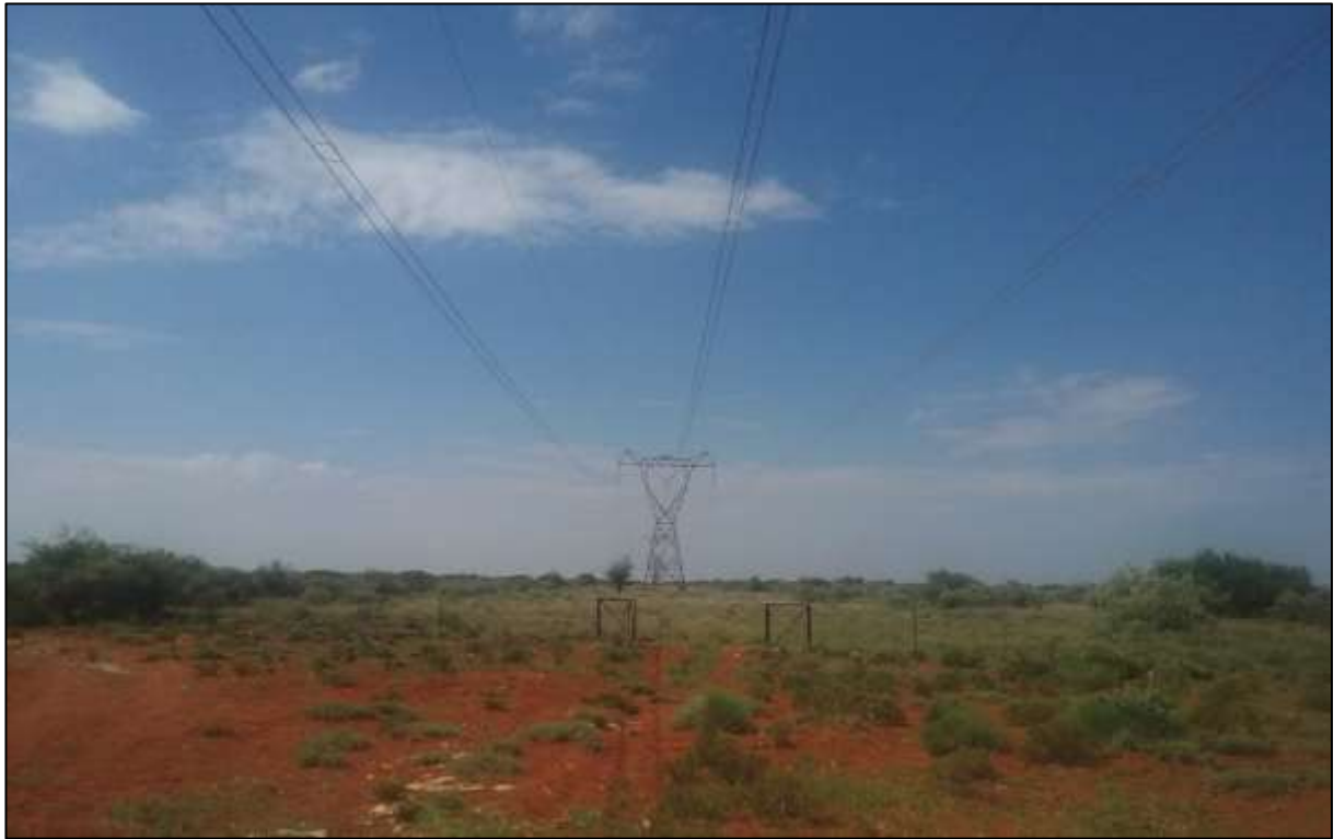
Figure 19: View from Photo 4 of the 400kV power line routed along the south-western boundary of the proposed site (Source: D. Holder Cape EAPrac 2018).
