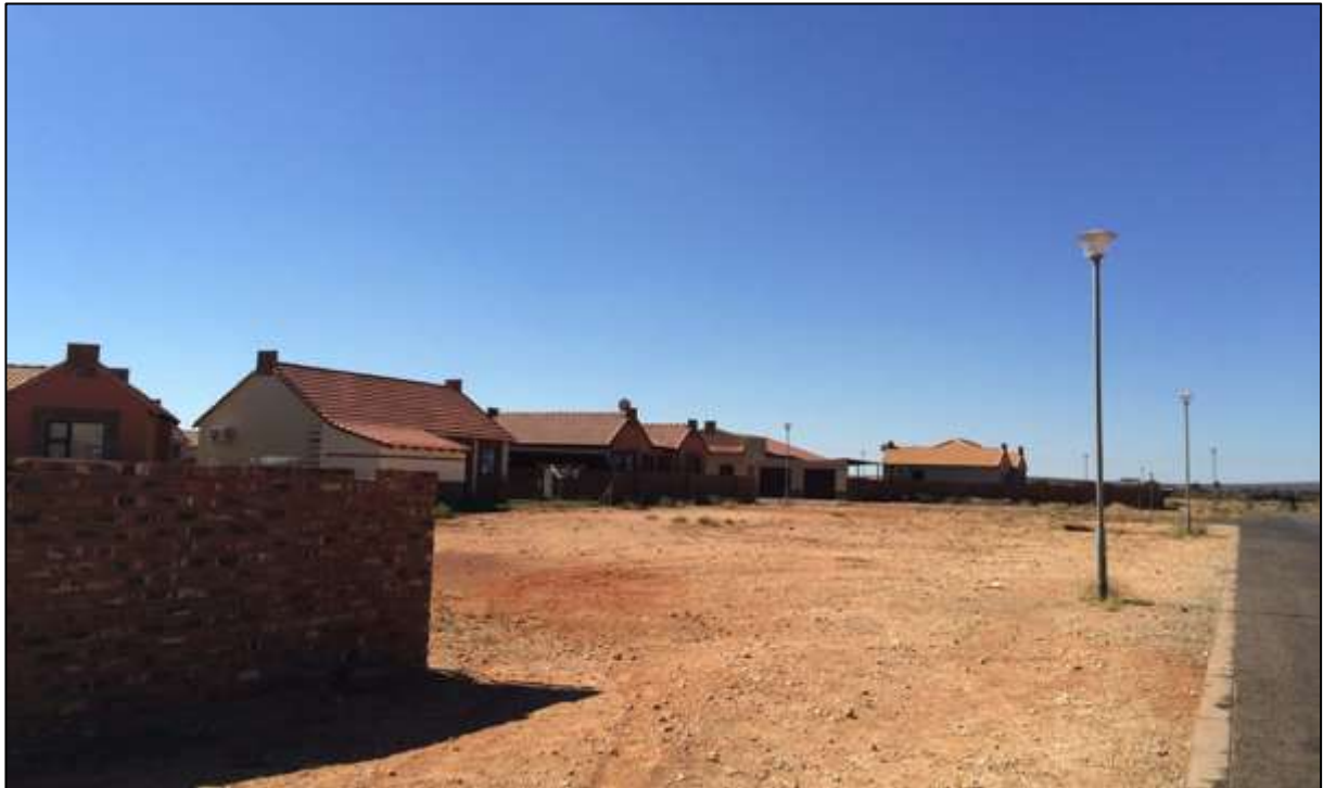
Figure 12: Photograph of the existing residential dwellings of the Bestwood estate.
