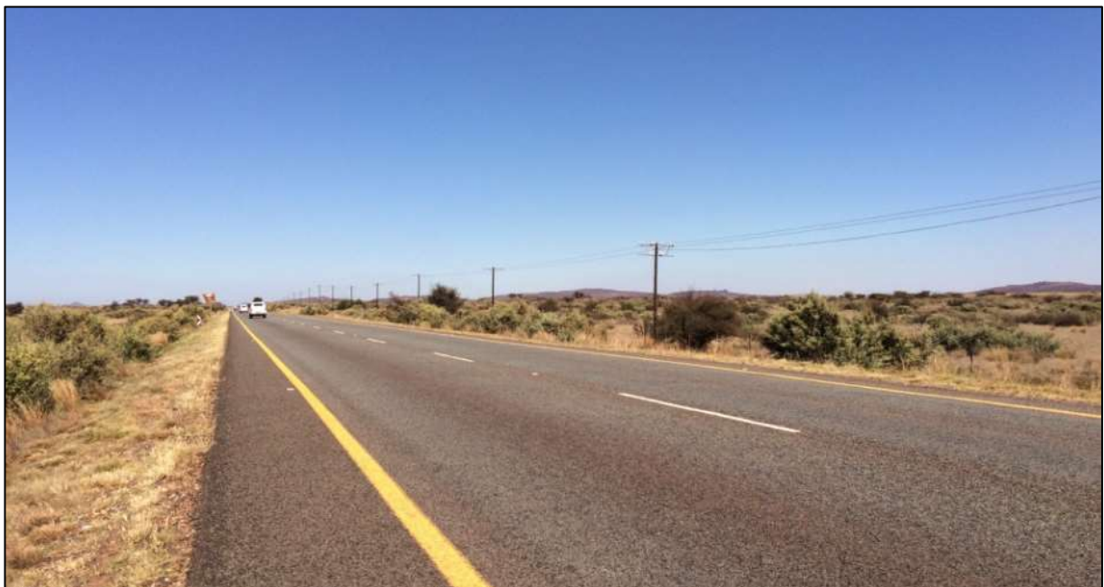
Figure 22: View south from Photo 7 showing the N14 national road crossing point.
