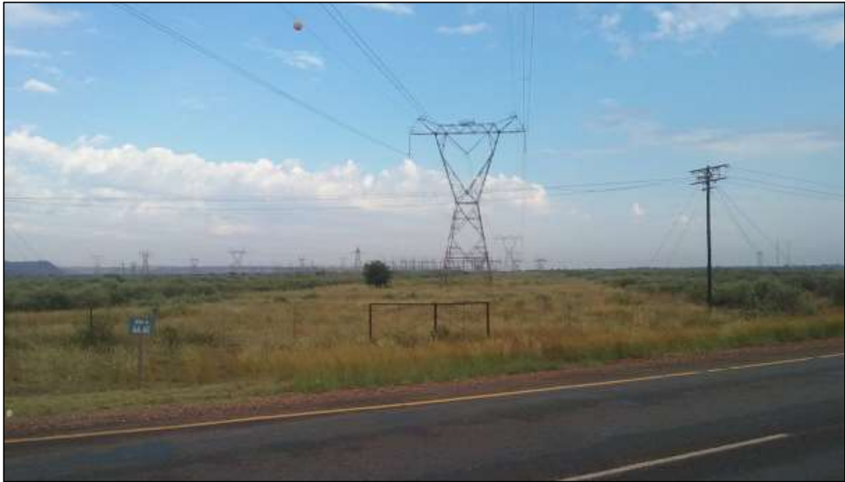
Figure 13: Photograph of the Ferrum Substation and 400kV powerlines leading to the substation (Source: D. Holder Cape EAPrac 2018).
