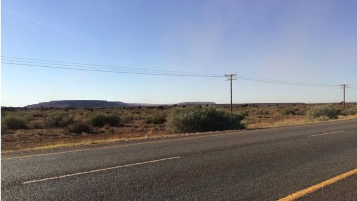
Figure 28: View west from Photo 9 location of the proposed 132kV power line crossing of the N14 with the Sishen Waste Rock Dumps located in the background.
