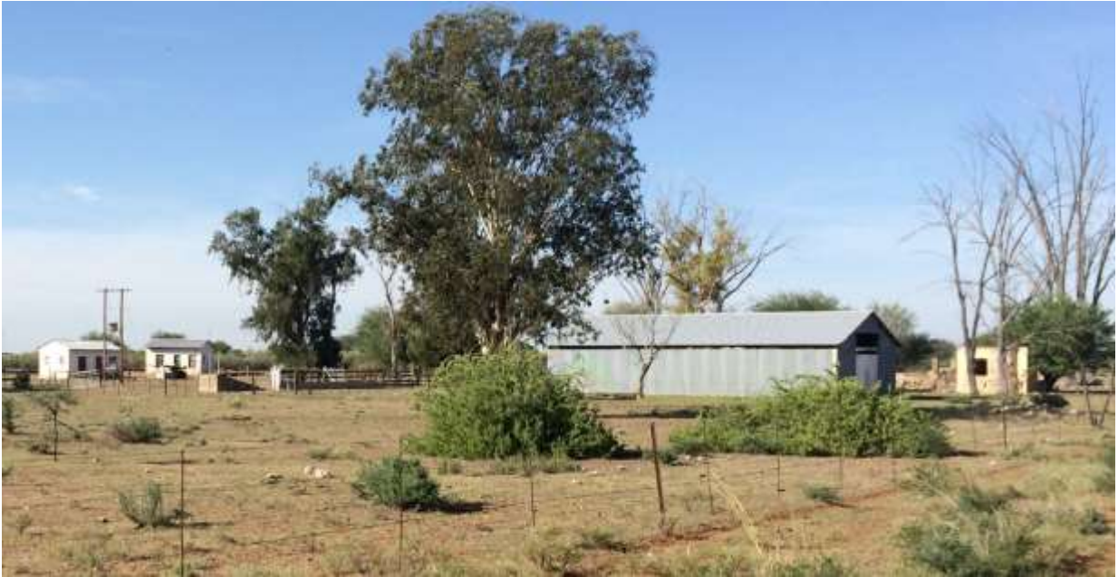
Figure 21: Photograph 2 in a southerly direction of some of the existing agricultural buildings found on the proposed site (non development area).
