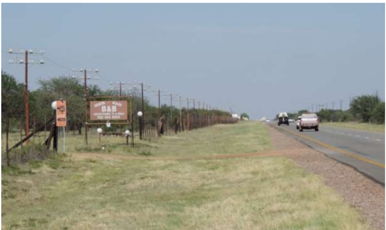
Figure 13: Photograph of one of the three tourist lodges located along the N14 National Road.
