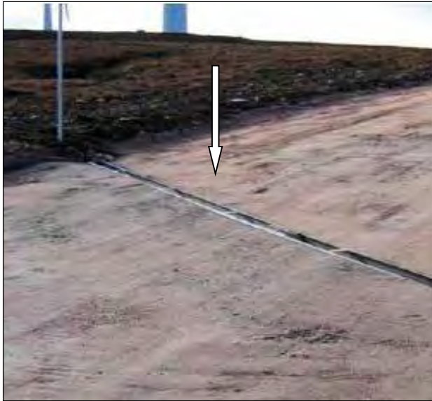
Figure 2-3: Cross drains under the Internal Roads
