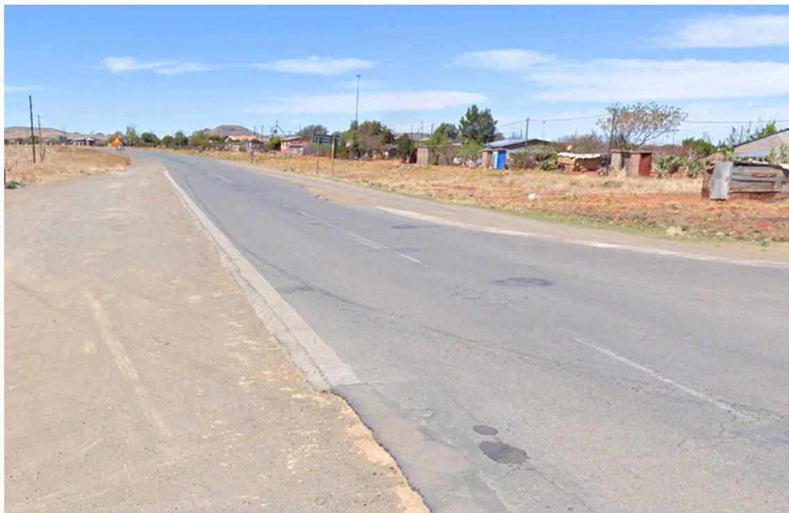
Figure 4-6: Sight distance on R48 in an eastern direction from S572
