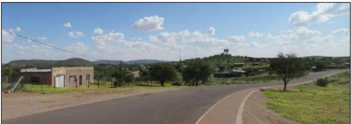
Photograph 3.2: Houses in Soverby seen from the main road through the settlement
