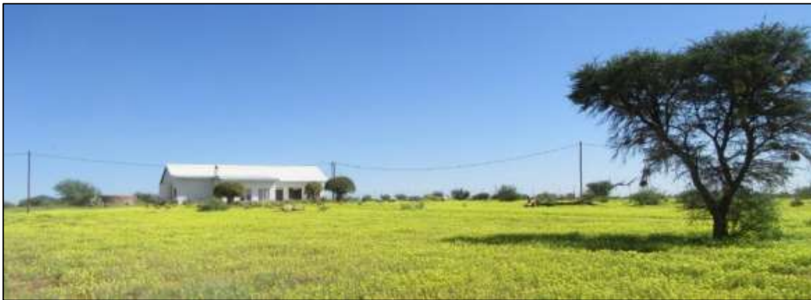
Photograph 3.14: Old farm school building located just to the north of the Geel Kop rail siding
