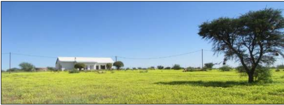
Photograph 3.14: Old farm school building located just to the north of the Geel Kop rail siding
