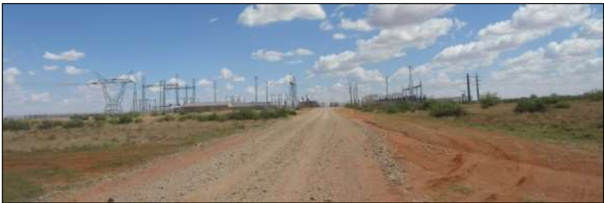
Photograph 3.11: Eskom's Upington MTS substation off the D3276 gravel road
