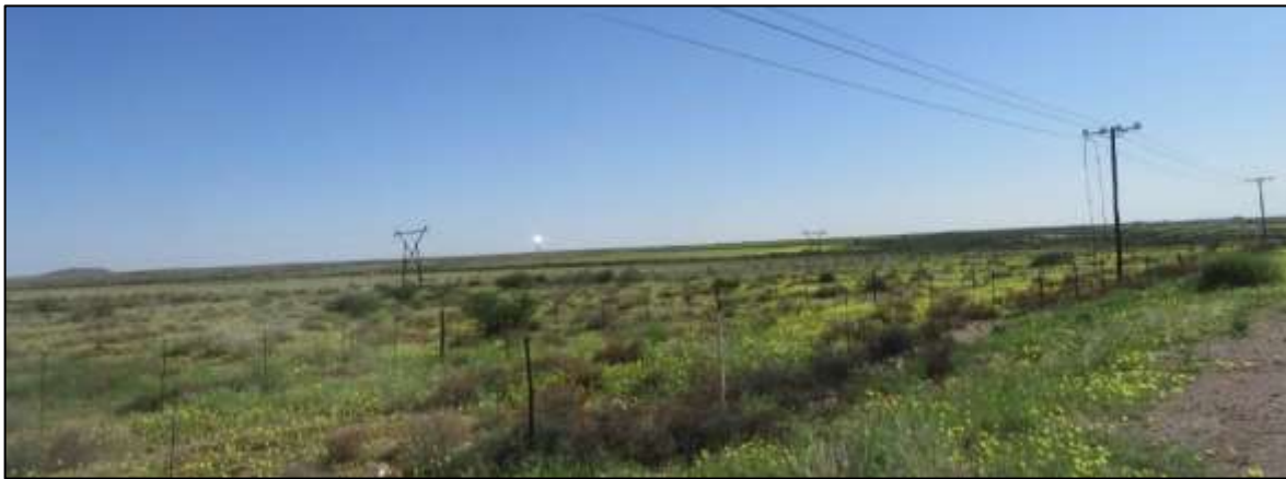
Photograph 3.10: Existing Eskom and Telkom lines located to the north of the N14
