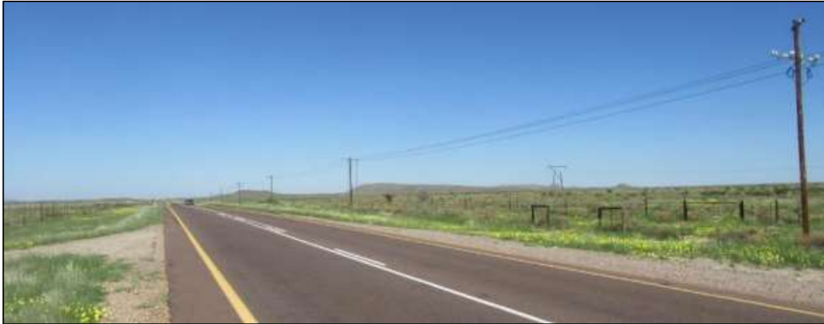
Photograph 3.1: N14, looking west (towards) Keimoes. The entrance road to the southern portion of RE Geel Kop Farm No 456 is visible on the left
