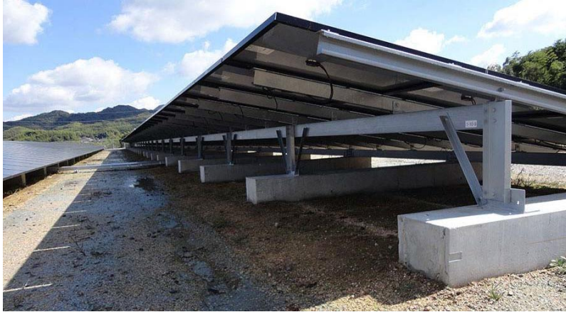
Figure 5: Cast Concrete Foundation (Solar Power Plant Business, 2013)
