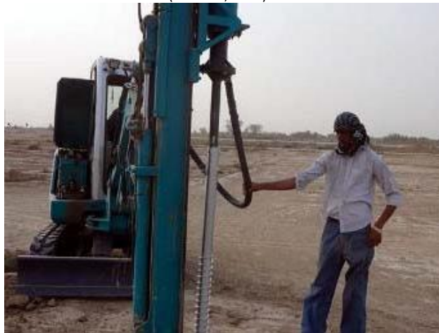
Figure 7: Ground Screw (PV MAGAZINE, 2014)
