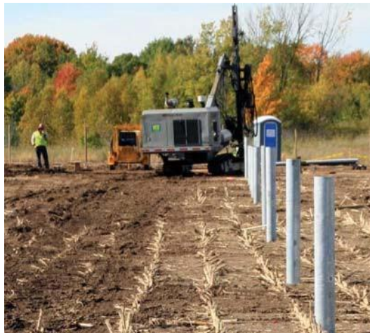
Figure 6: Driven/ Rammed Steel Pile (SolarPro, 2010)
