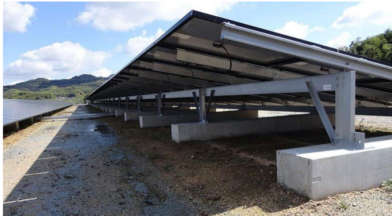
Figure 5: Cast Concrete Foundation (Solar Power Plant Business, 2013)
