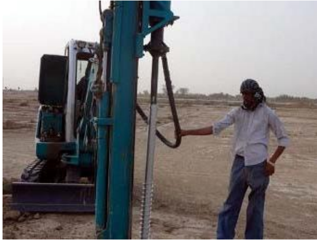
Figure 7: Ground Screw (PV MAGAZINE, 2014)
