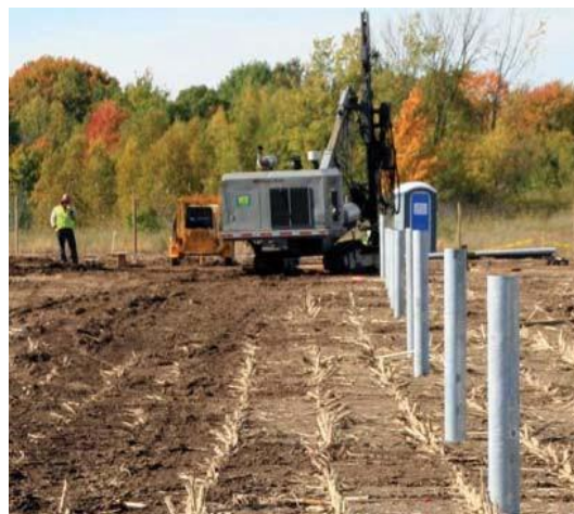
Figure 6: Driven/ Rammed Steel Pile (SolarPro, 2010)
