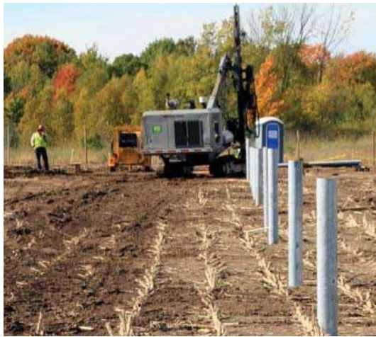
Figure 7: Driven/Rammed Steel Pile (SolarPro, 2010)
