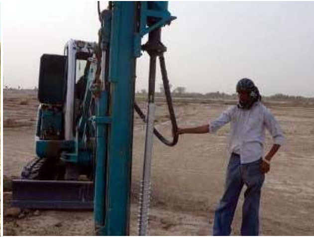
Figure 8: Ground Screw (PV MAGAZINE, 2014)
