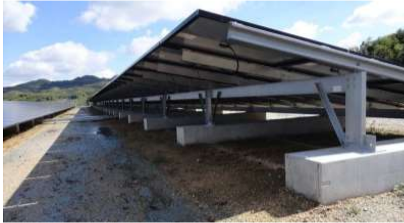
Figure 6: Cast Concrete Foundation (Solar Power Plant Business, 2013)
