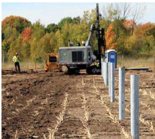
Figure 7: Driven/ Rammed Steel Pile (SolarPro, 2010)
