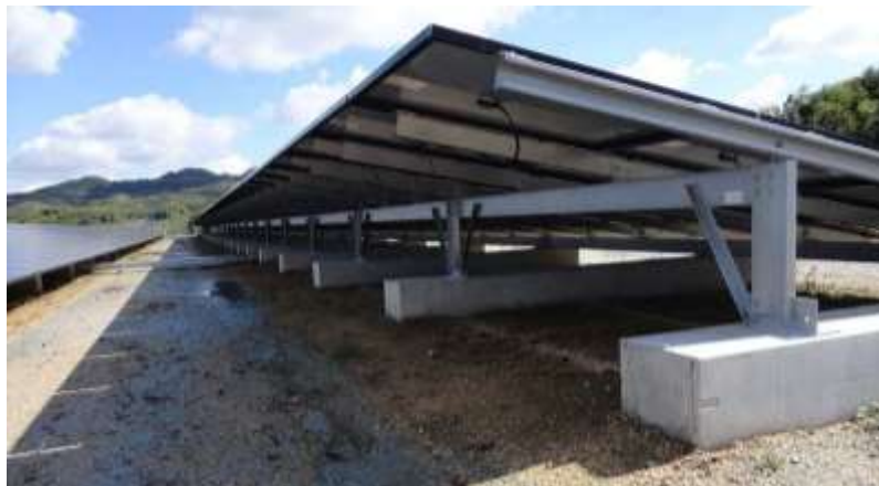
Figure 6: Cast Concrete Foundation (Solar Power Plant Business, 2013)
