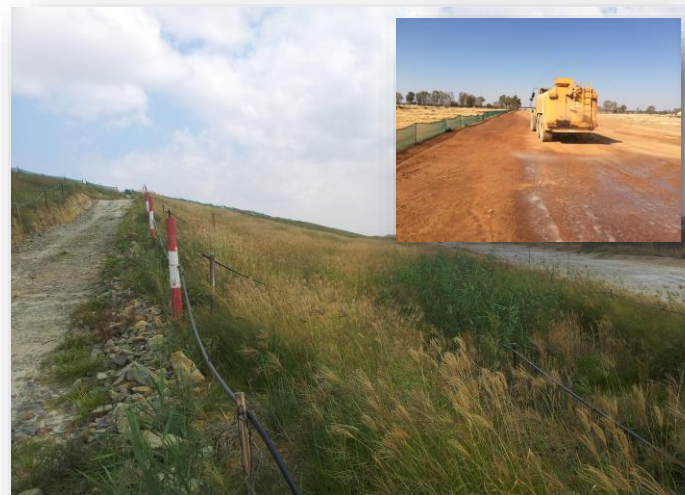
Tailings Dam Grassing
