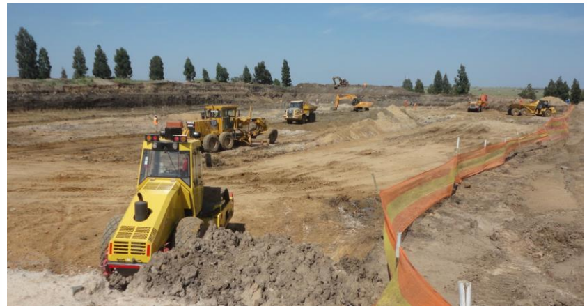
Additional water containment dam - Kareerand
