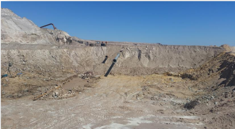
Reclamation Site - Containment
