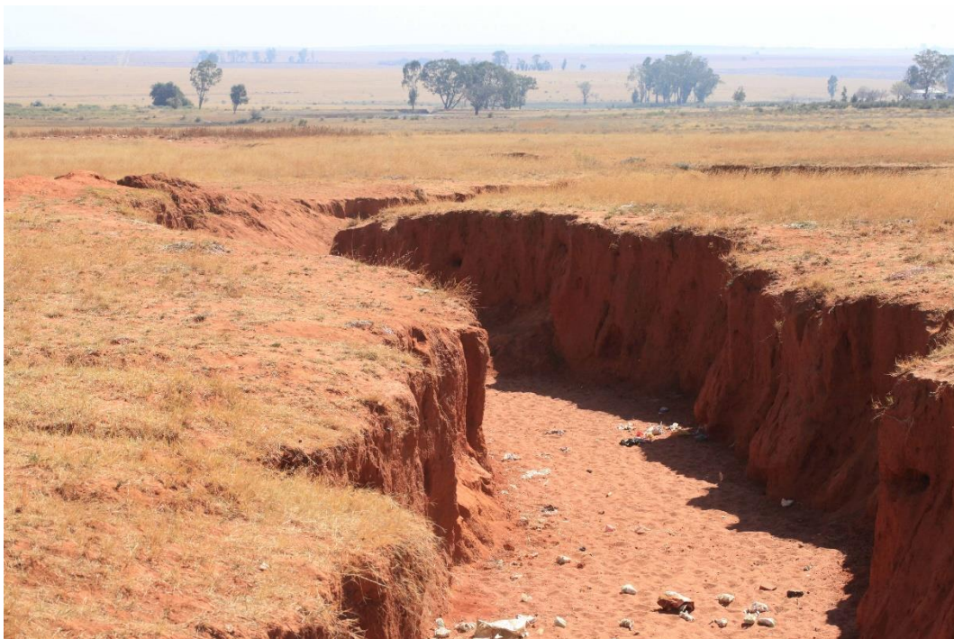
Photo 2 Erosion at the site caused by stormwater and exposed soil. Photo: R.F. Terblanche
