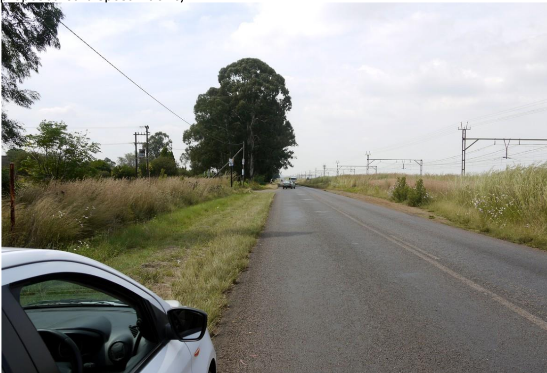
Plate 13, The R555 – The existing railway largely screens views of the existing mine stockpiles and is likely to also provide screening for the proposed co-disposal facility from the majority of the road.
