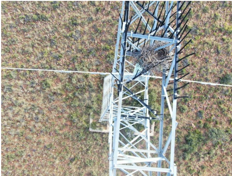
Figure 8: Jackal Buzzard nest on high voltage powerline pylon in the Study Area.
