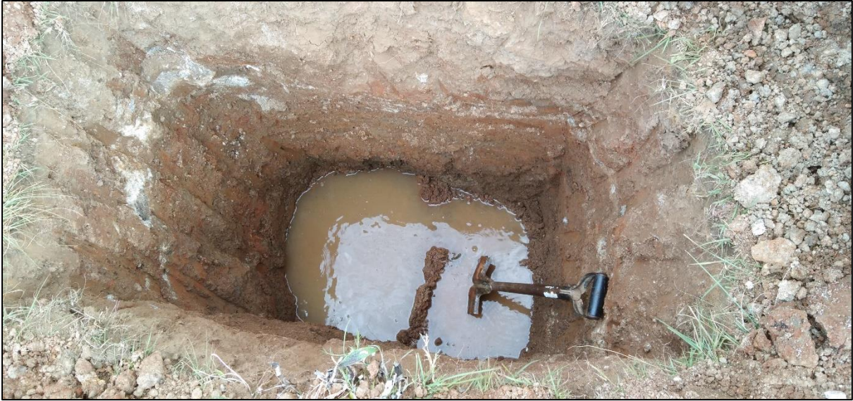
Photograph 8: Water Seepage and Material Encountered in TP205
