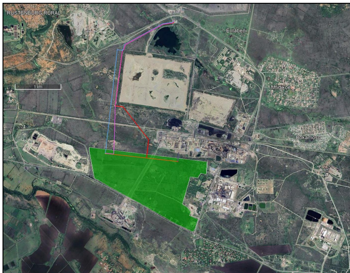
Figure 6: Aerial view of the proposed SRPM PV facility.
