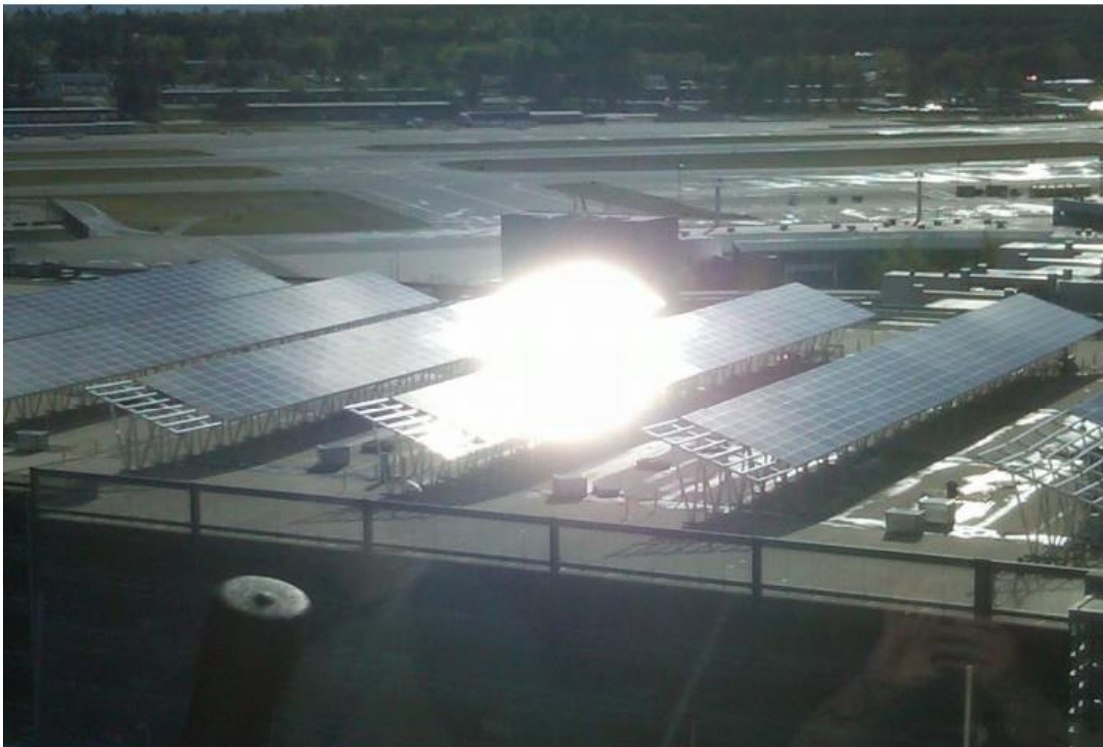
Plate 13 - Glare experienced in the Control Tower at Boston Regional Airport from an adjacent PV array
