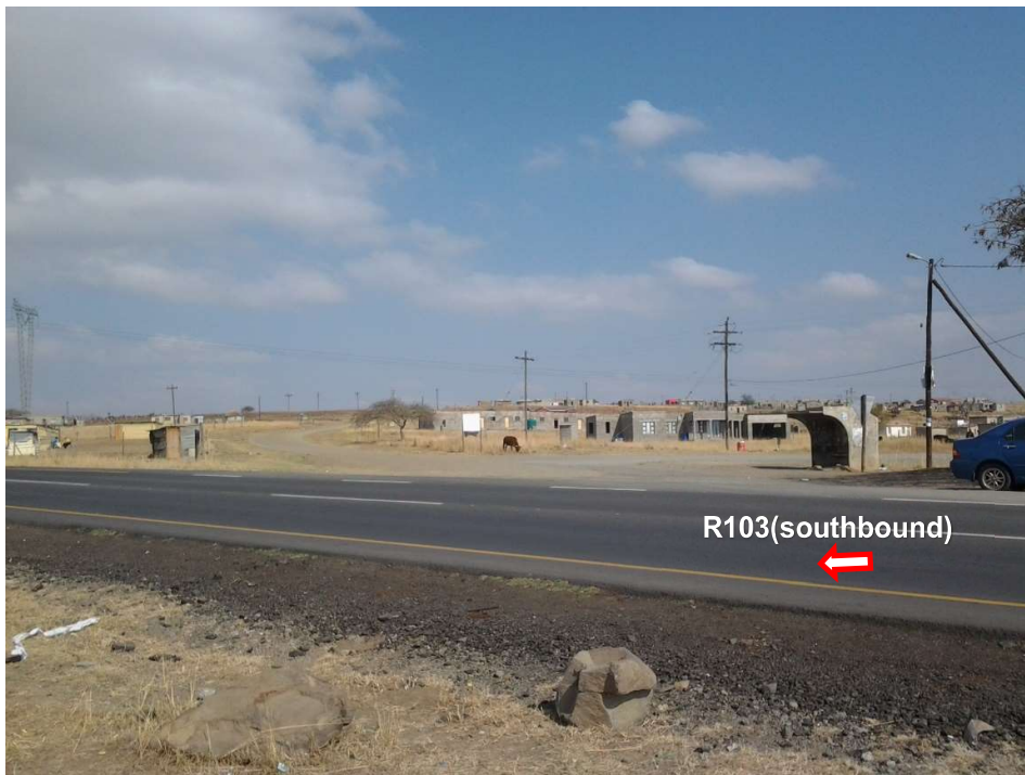
Image 2: Road conditions on intersection of R103 and D637 (Intersection 2)
