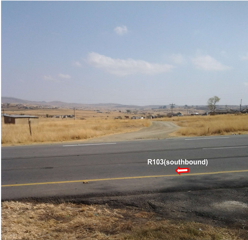
Image 1: Road conditions on intersection of R103 and Unnamed Road A (Intersection 1)
