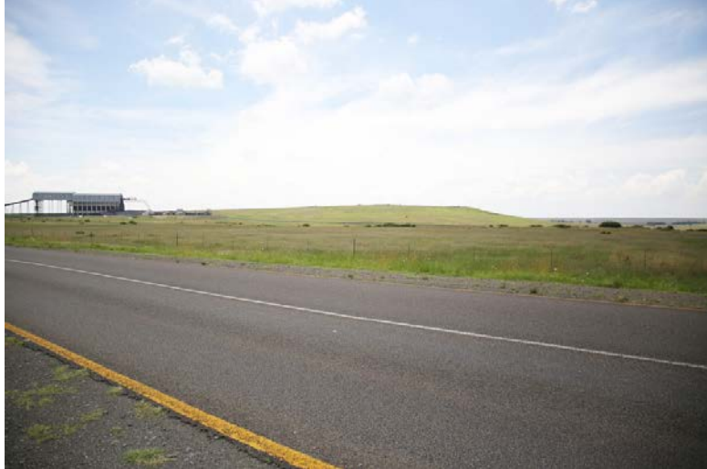
Route along the Impumelelo conveyor belt
