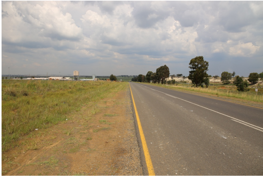
Zandfontein substation site on left of Brendon Village road.
