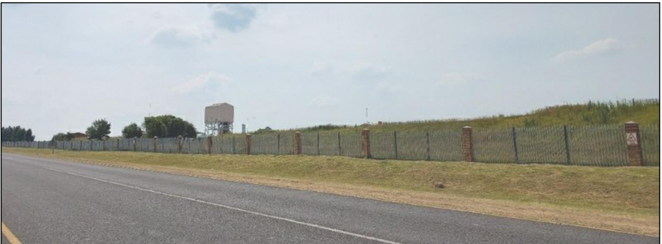
Figure 15: View along the northernmost part of the corridor where it runs adjacent to a mine.
