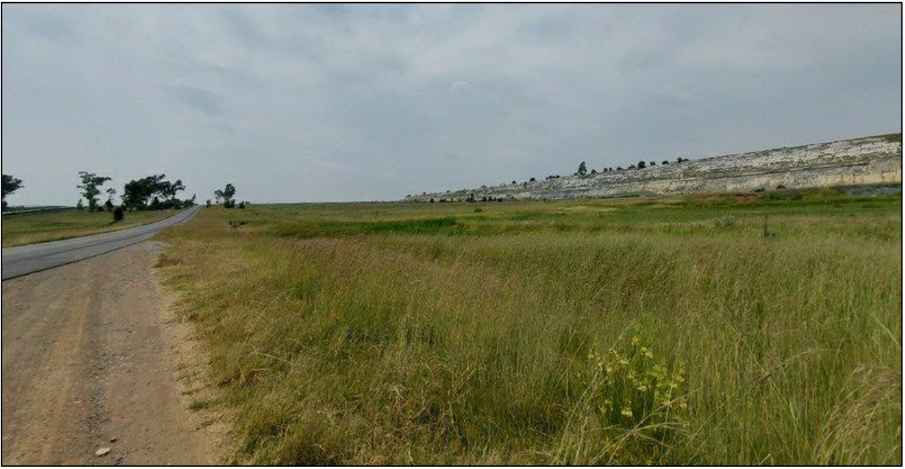
Figure 14: View east along the grid corridor where it follows a road leading off the R547. A mine dump lies to the right.
