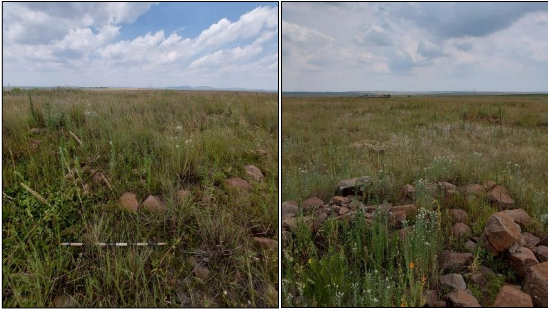
Figures 32 – 27: General site conditions at IM011 showing the remains of stone walling scattered across the low overgrown hill.
