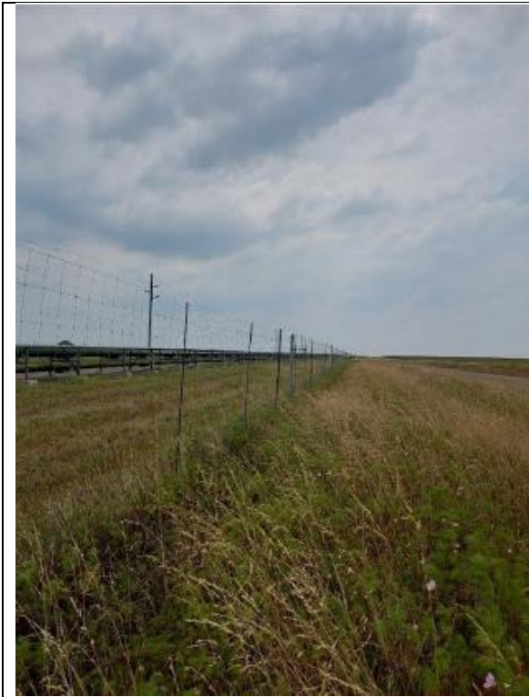
Figure 5A – general view of undulating lands covered with deep soils and secondary grassland. Conveyor belt along the left.
