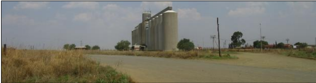
Photograph 3.5: Trichardt silos at the southern entrance to Trichardt.
