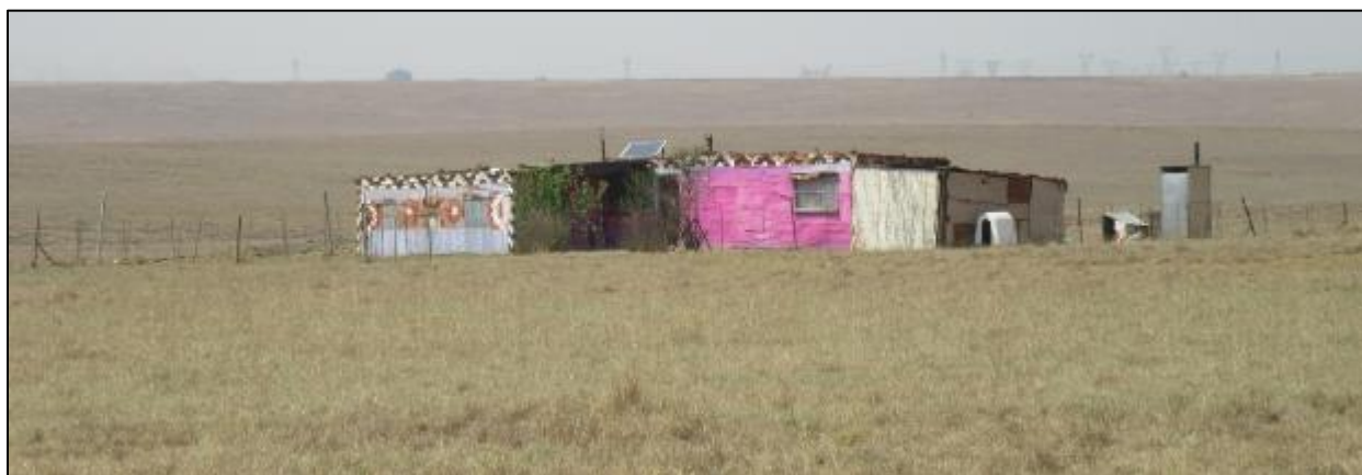
Photograph 3.10: Worker's dwelling on Vantondershoek 317/12
