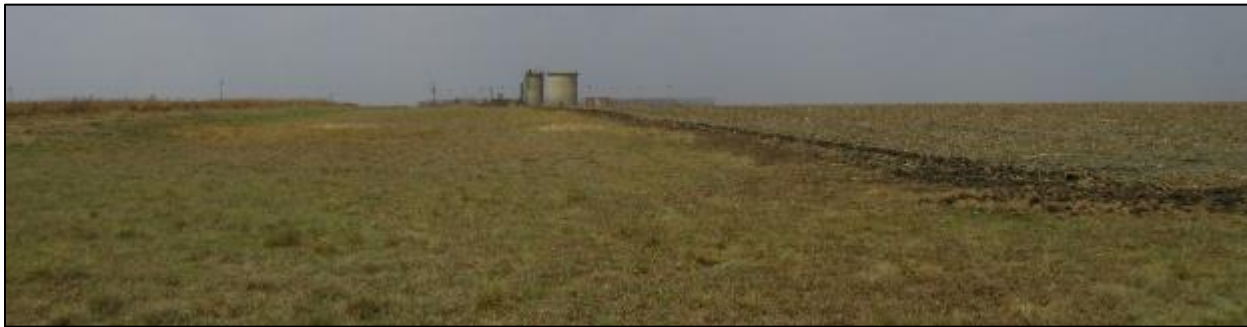
Photograph 3.3: Buried coal conveyor belt on Brandwacht 316/3
