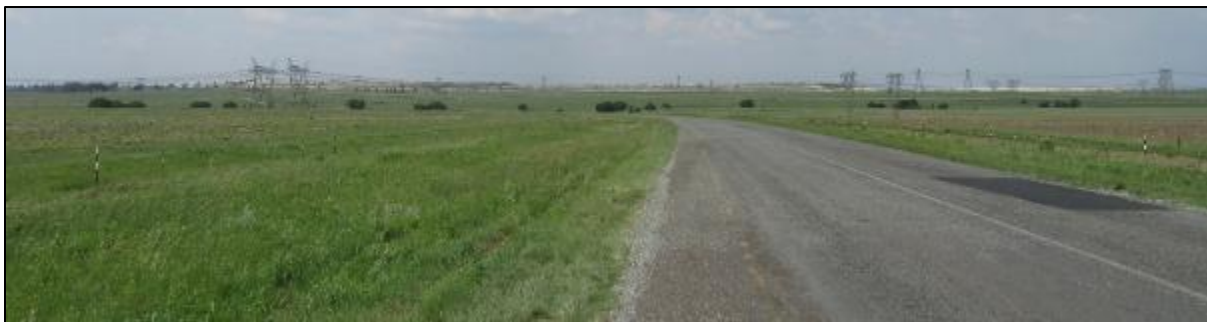
Photograph 3.25: 400 kV corridor crossing R547N in the northern portion of Springbokdraai 277/3, looking north.
