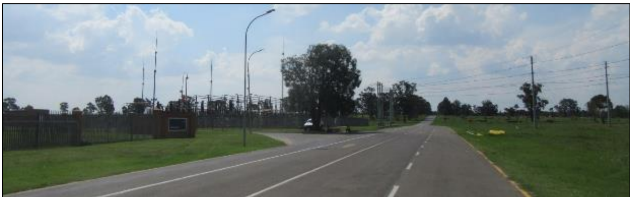
Photograph 3.23: Entrance to SASOL's Simunye Shaft premises and 132 kV lines entering Zandfontein substation, seen from the access road (S) to Brendan Village (distant background).
