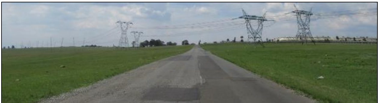
Photograph 3.19: Overhead lines to Leslie mine crossing the R547N on Zandfontein 130/9 (Evander)
