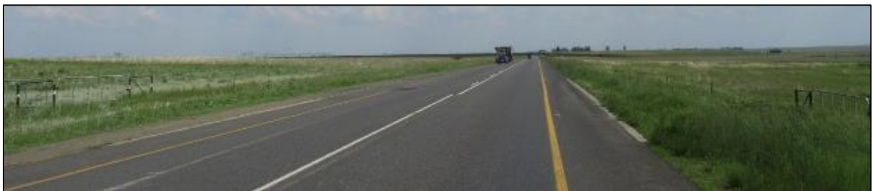
Photograph 3.29: Portion of the R50 between Vaalbank and Springbokdraai flanked by rangeland and fields used for dryland cropping (left middle ground), looking north.
