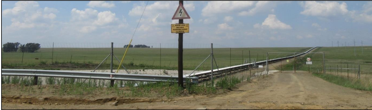
Photograph 3.16: Coal conveyor line from Impumelelo mine to SASOL Secunda
