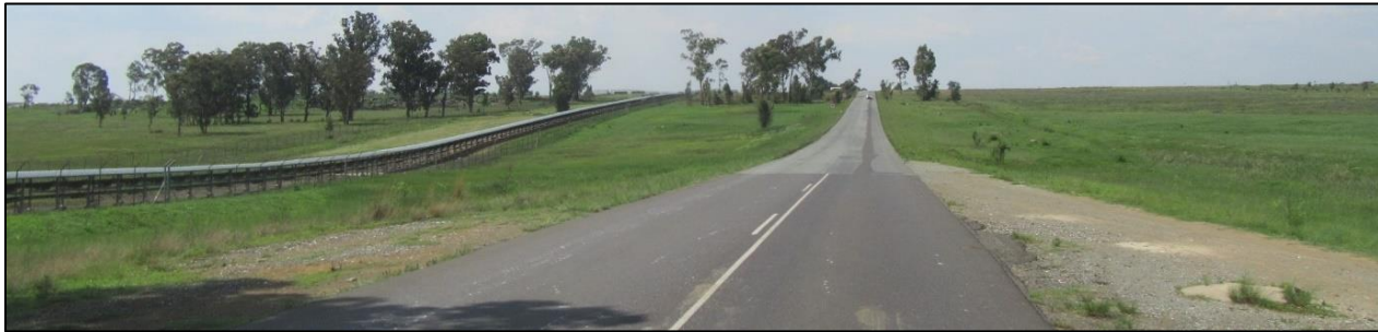
Photograph 3.17: Coal conveyor line portion located to the west of the R547N looking north
