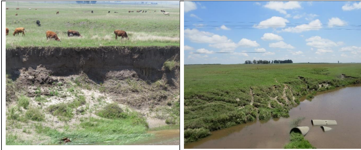
Figure 18: Indicating some of the impacts recorded on site. Including mining, erosion, grazing and broken infrastructure
