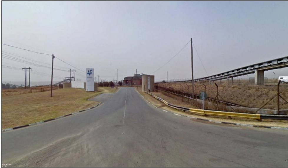
Figure 12: Substation and coal conveyor adjacent to the Riaan Rademan Training Academy (Source: Google Earth 2022)
