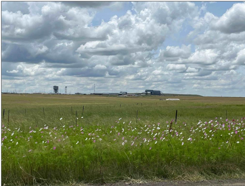
Figure 7: View of Impumelelo Mine in the south-western sector of the study area
