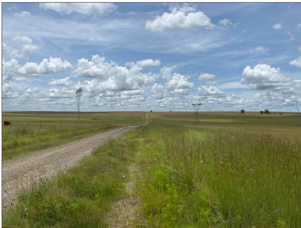
Figure 8: High voltage powerlines traversing the southern sector of the study area.
