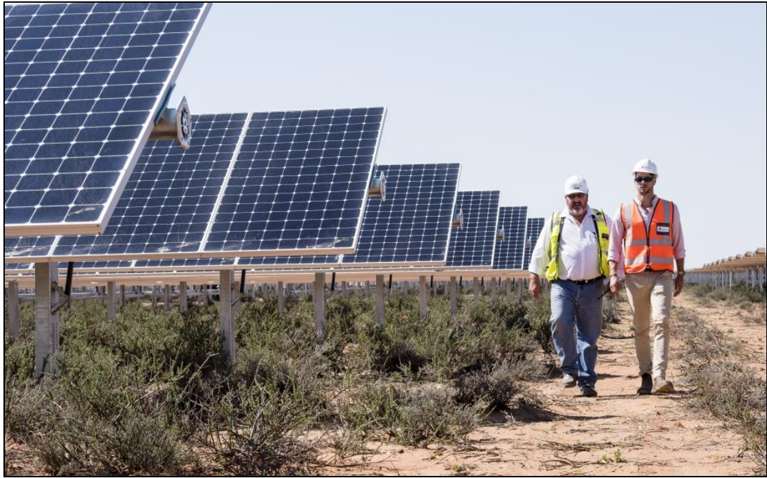
Figure 1: Photovoltaic (PV) solar panels. (Photo: SunPower Solar Power Plant-Prieska)
