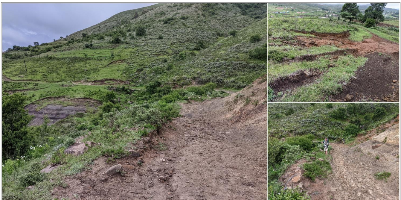
Figure 3 The site along the proposed road area
