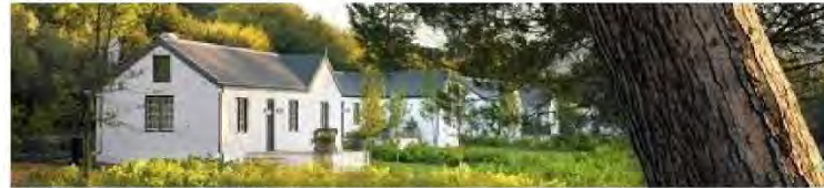
Example of rural free standing cottage - Werf cottages at Boschendal
