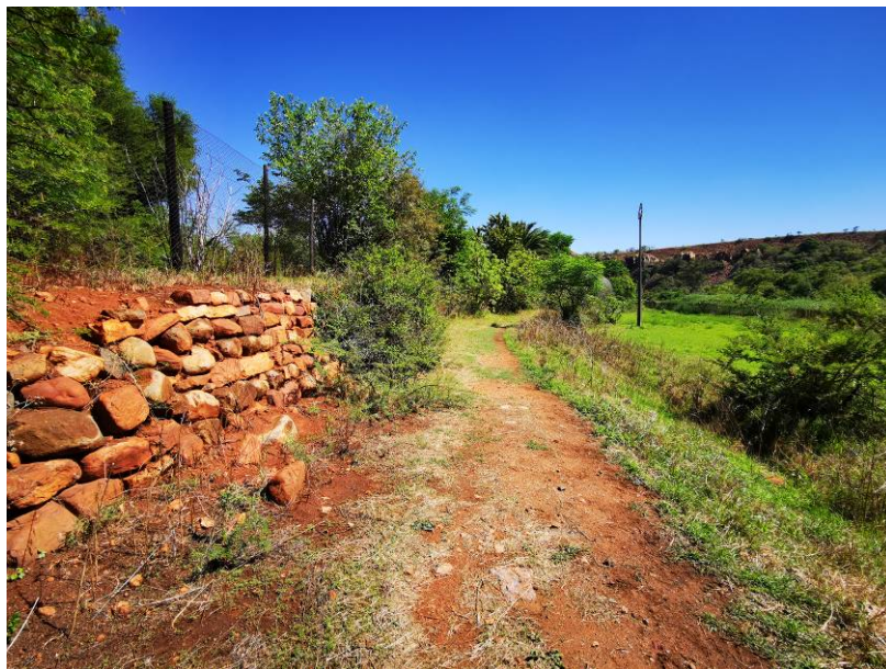
Figure 12: Dry stone terracing of CSF garden systems dating to 1970s and located outside project area.
