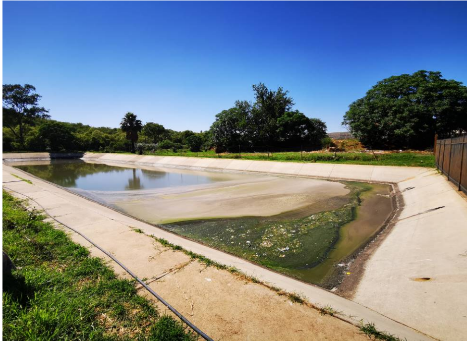
Figure 4: Pre-treatment facilities on the Grounds of the Baviaanspoort CSF.
