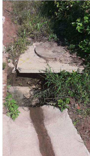
FIGURE 14: EXISTING STORMWATER INLET STRUCTURE
