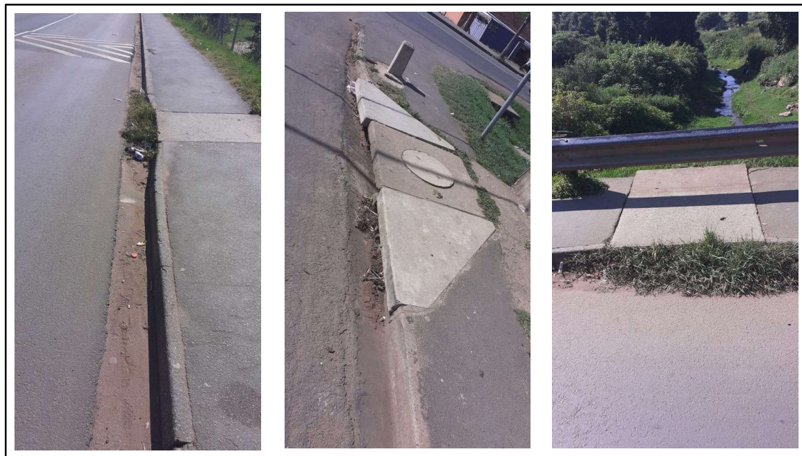
FIGURE 13: EXISTING STORMWATER KERB INLETS
