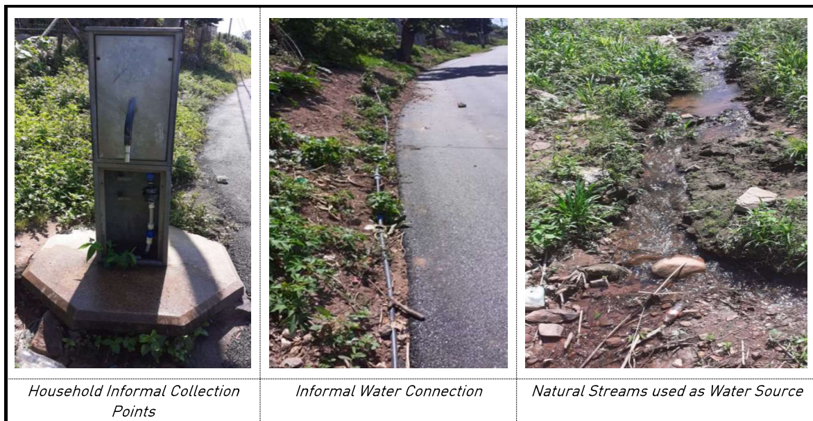
FIGURE 6: ACCESS OF WATER IN AMAOTI INFORMAL SETTLEMENT
